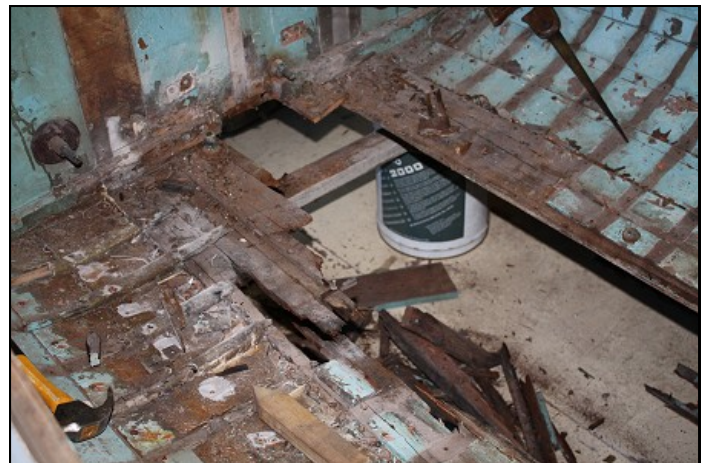
The extent of deterioration is obvious here . . .
