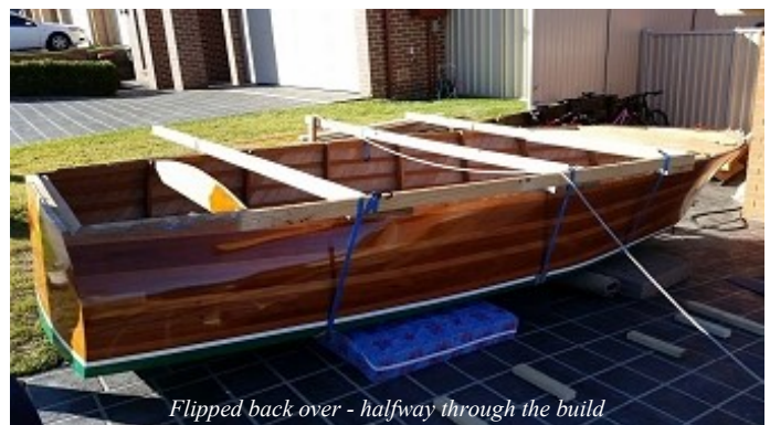
Using tie down straps to shape the timber to the complex curve of the boat
